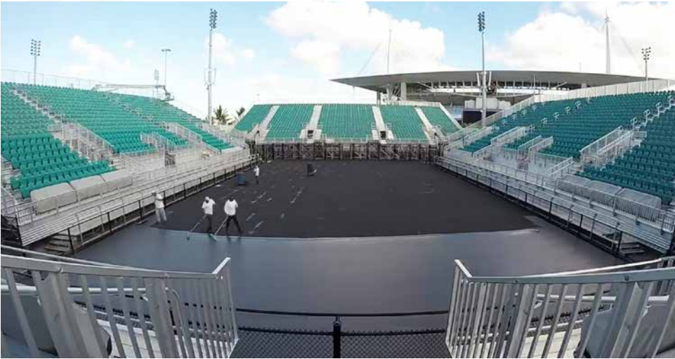
Applying the Laykold Resurfacer
