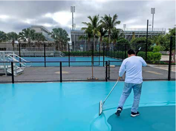
Applying the LM Topcoat
