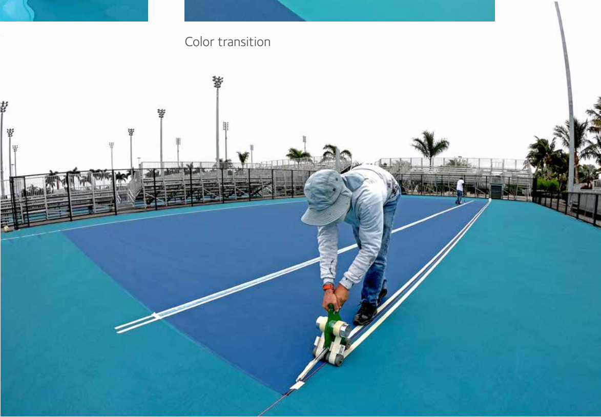
Taping in preparation for line paint
